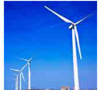
风力发电站 Wind power station
